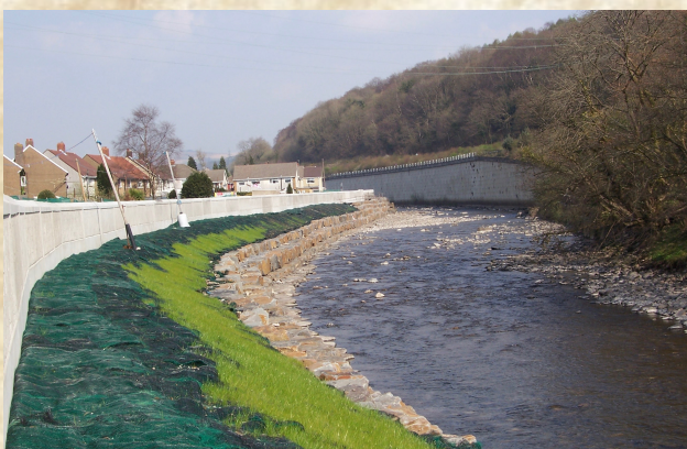
The Finished Glynneath Flood Alleviation Scheme
